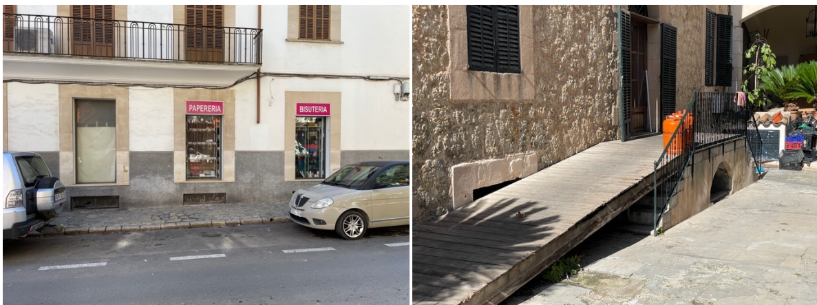
Figure 21. Cellar windows are observed occasionally along Gran Via Colom (Photos: Fekete, Inca, 26 Feb. 2025).
