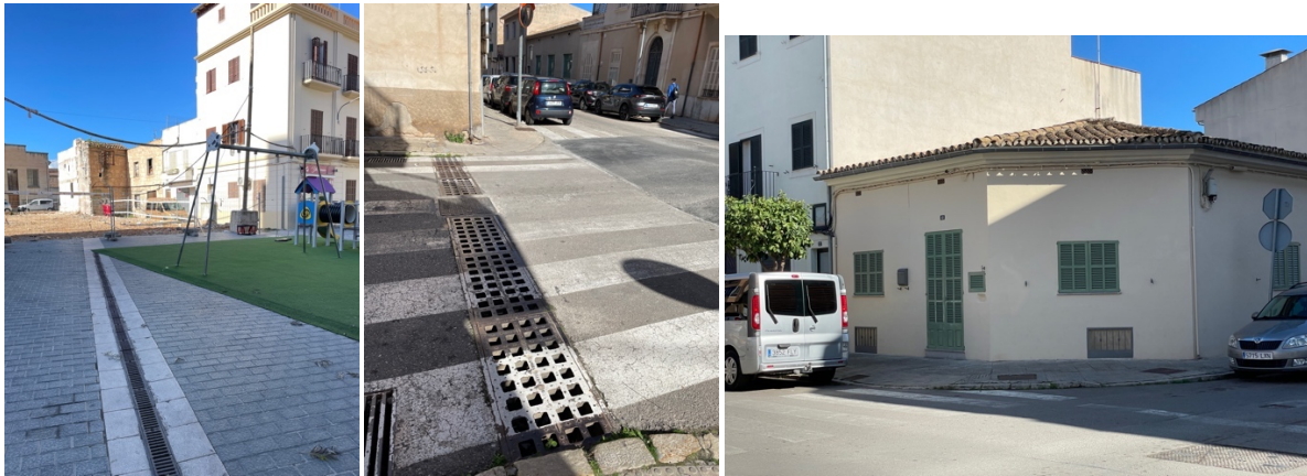
Figure 24. Road drainage examples at the Placa de la Quartera (left), and along the Carrer d'en Ramon Llull Beato (Photos: Fekete, Inca, 26 Feb. 2025).
