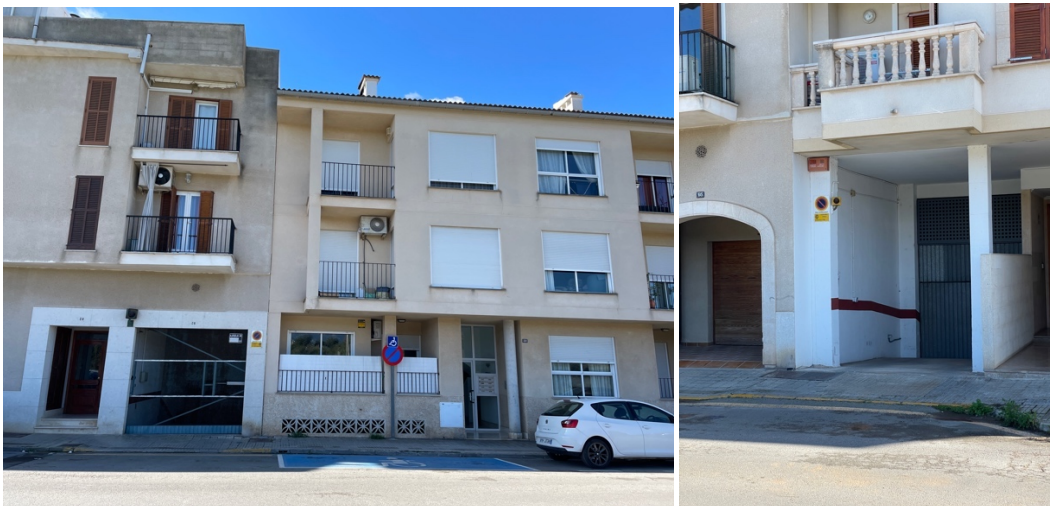
Figure 27. Basement windows and underground garage entries along the urban rim road Carrer de Mandrava (Photos: Fekete, Inca, 26 Feb. 2025).
