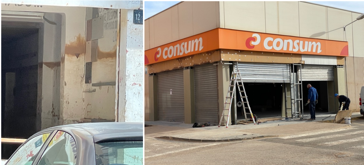
Fig. 3 Flood level on a garage wall and renovation work on a supermarket in Paiporta (Fekete, 8.1.2025)
