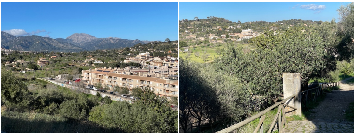
Figure 29. Additional entry points of torrents into the city of Inca from the north, picture taken from the Carrer dels Canonges Garau; and entrance to the Parc de Serral de ses Monges (Photos: Fekete, Inca, 26 Feb. 2025).
