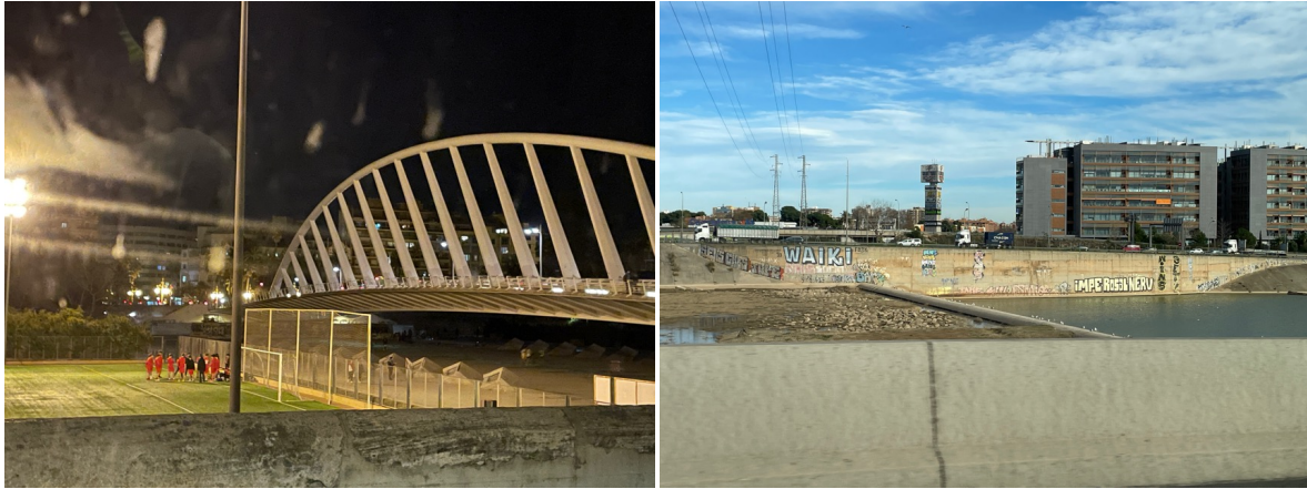
Fig. 2 Left image Modern buildings and sports facilities in the former riverbed of the River Turia through the city of Valencia. Right image: Turia flood channel after the detour in the south of the city (Fekete, 8.1.2025)
