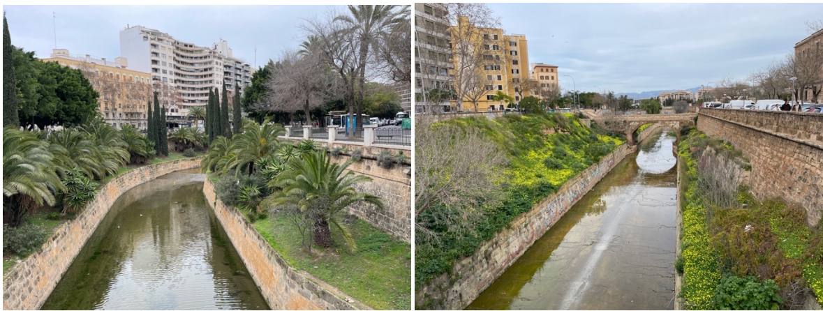
Figure 8. Diverted canal of the Sa Riera River with concrete bed and walls in Palma (Photos: Fekete, Palma, 25 Feb. 2025).
