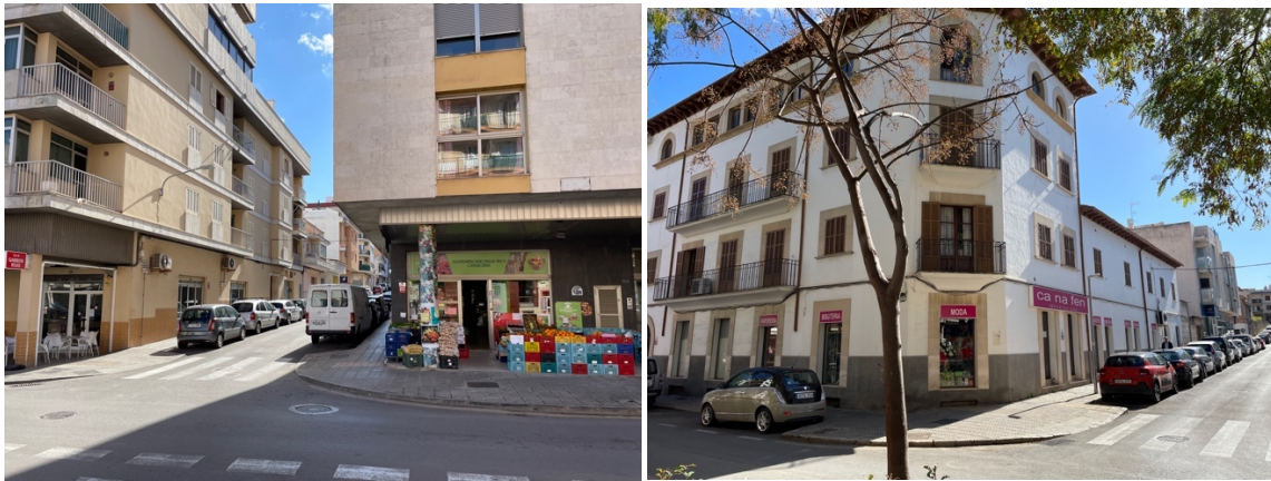
Figure 22. Inclining roads left and right of the former river bed (Photos: Fekete, Inca, 26 Feb. 2025).
